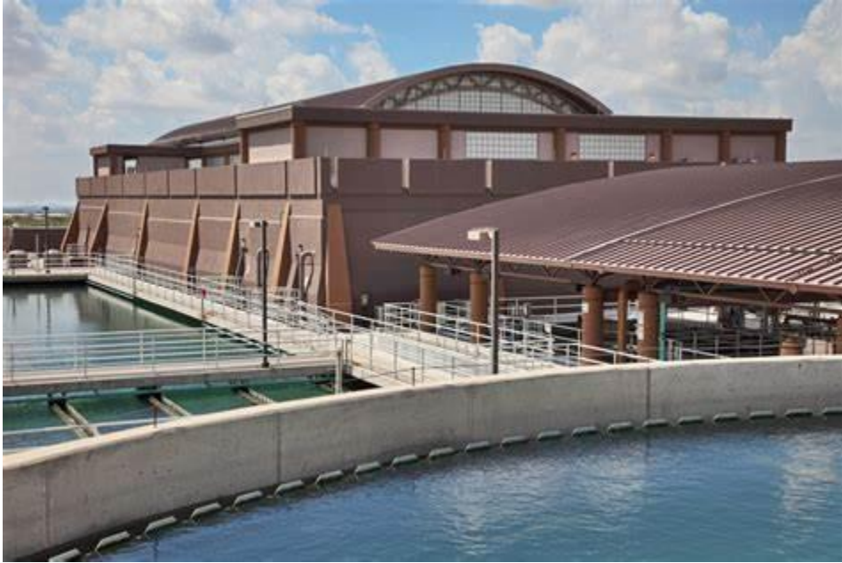
2011 CAP Water Treatment Plant Expansion
